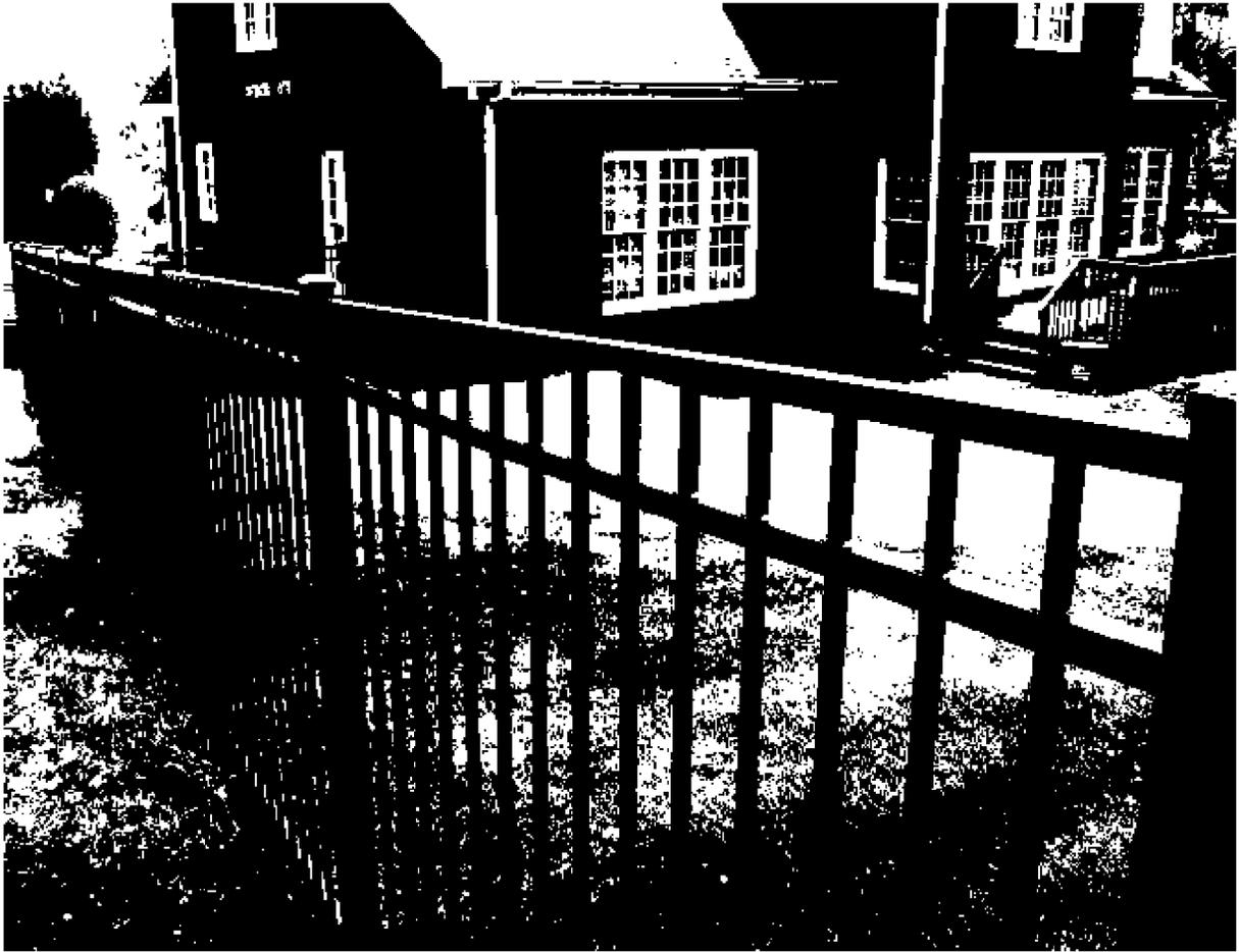
Type B upgraded Iron fencing – Iron fencing is to be 48” tall with 3” x 3” posts spaced 8’ on center. Pickets are to be 4” apart from one another. Per the image above the wooden fencing will slope down to meet the top elevation of iron fencing. All Iron fencing will be from the same manufacturer, and of the same color.
